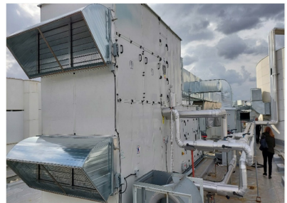
Picture 5. Replacement of AHU-18 and AHU-19 with heat recovery air handling units (Before vs After)
