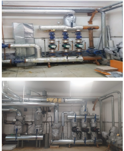
Picture 6. Circulation Pumps Replacement (Before vs After)
