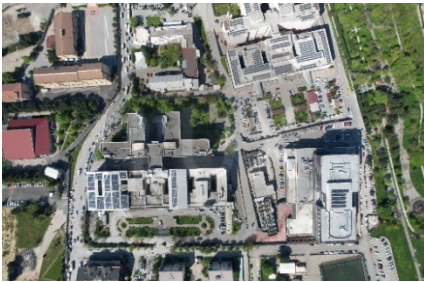
Picture 9. Rooftop solar photovoltaics (PV)
