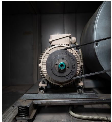
Picture 4. Belt and Pulley (Cogged V-Belt)
